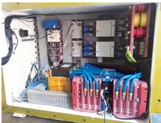
Feeder Breaker Controller installation
